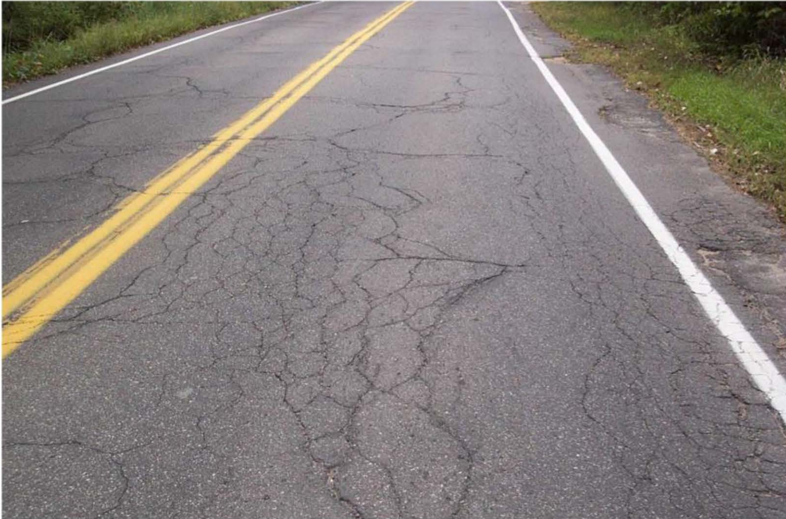
Figure 20. Alligator Cracking
